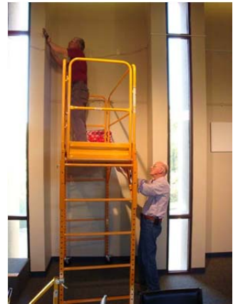
Ron Pasch and Paul Adler installing the telecoil.
